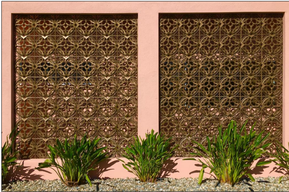
Shown here is the larger of the two walls which consists of a pair of AGU arrays. The AGUs elegantly screen the residence from the morning sun.
