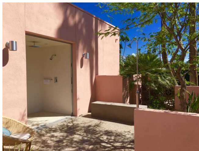
While the 2016 bathroom modification (and associated wall) impacted the original fabric, the change is both sympathetic and reversible (see Section 7 “Integrity Analysis”).
