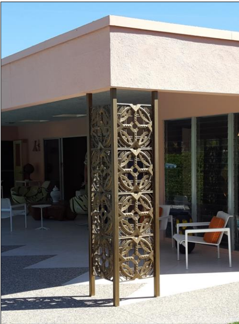
Steel 2"x2" support columns and AGUs.
